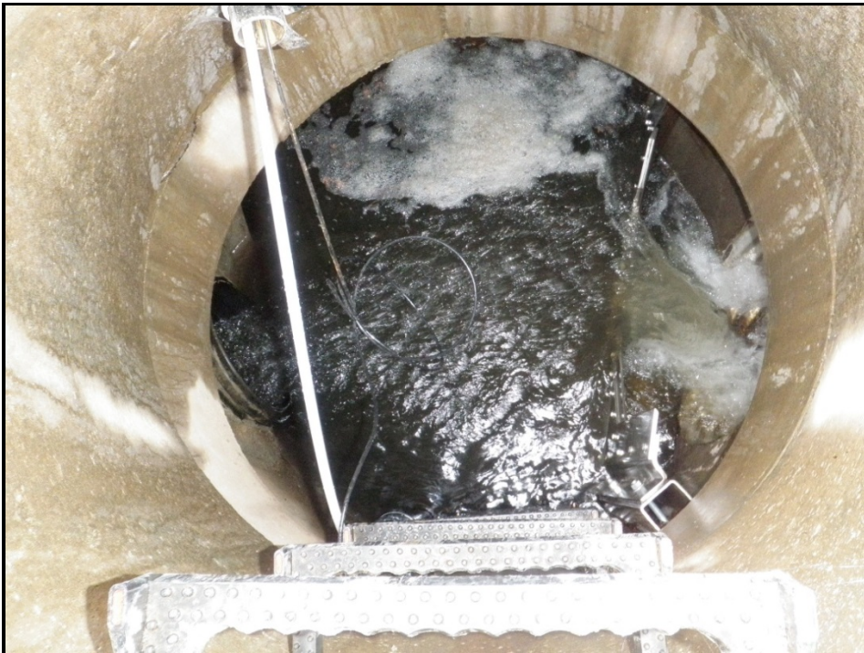
Figure 4 View down HDR's stormwater manhole with large v-notch weir on right side
